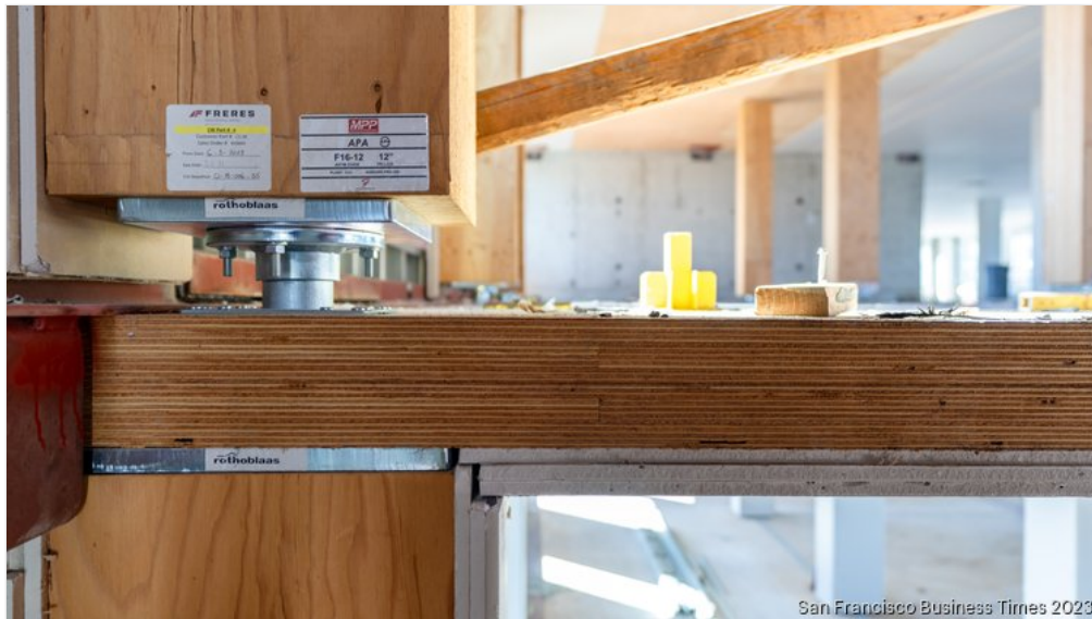
A floor currently under construction by oWow showing the thickness of the floor using mass timber in downtown Oakland, Calif. on September 7, 2023.
