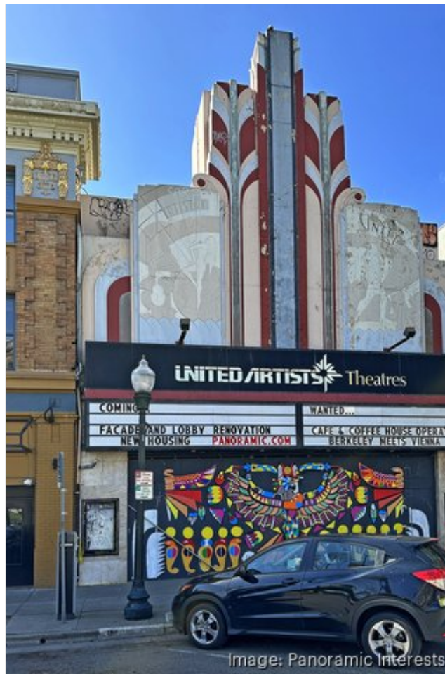
The current facade of 2274 Shattuck Ave.
