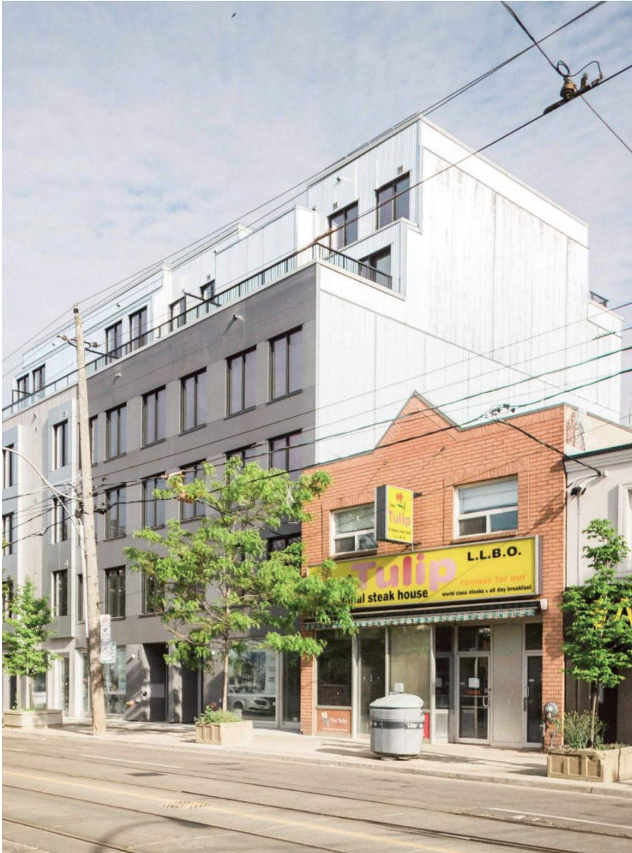
Photo Courtesy of Assembly Corp.
