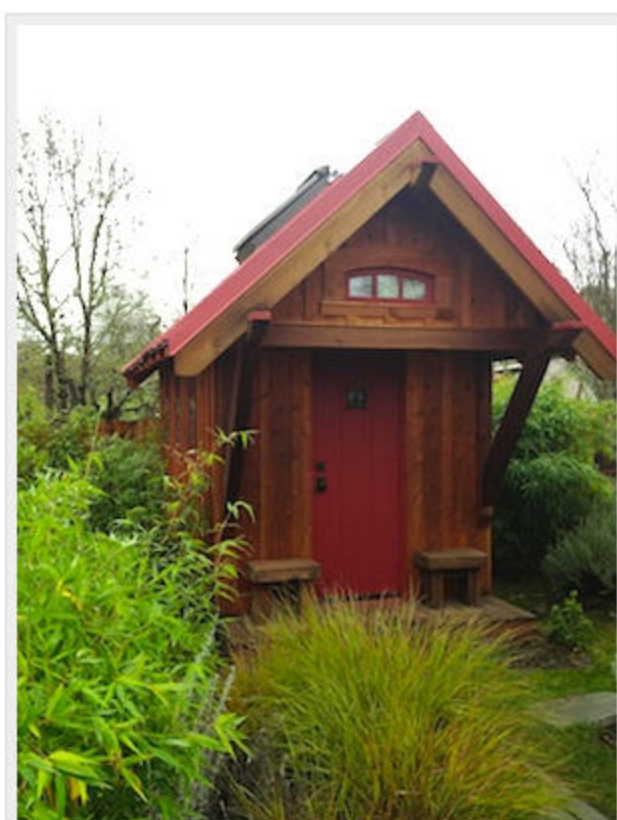
Jay Shafer's 106-square-foot tiny home in Sebastopol, California.
