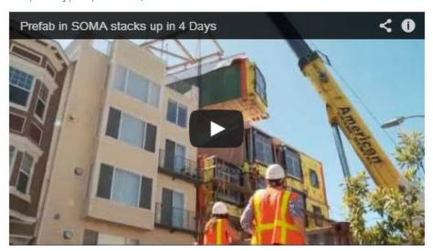
We also came across the above video that shows some of 38 Harriet's prefab construction process. By using offsite construction, they were able to turn an uncovered foundation into a four story building in a mere three days.
