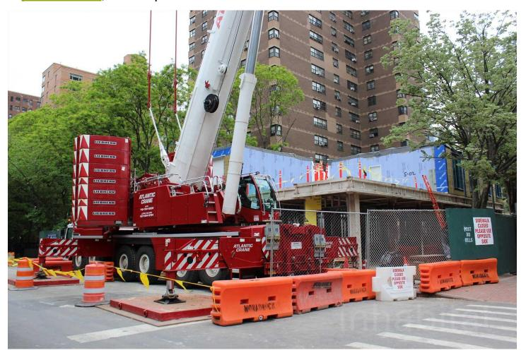
The modular units that make up the development were fabricated by Monadnock sister company <u>Capsys</u> at the Brooklyn Navy Yard and will be transported to the construction site gradually over the next few weeks. The first modules are already in place.
