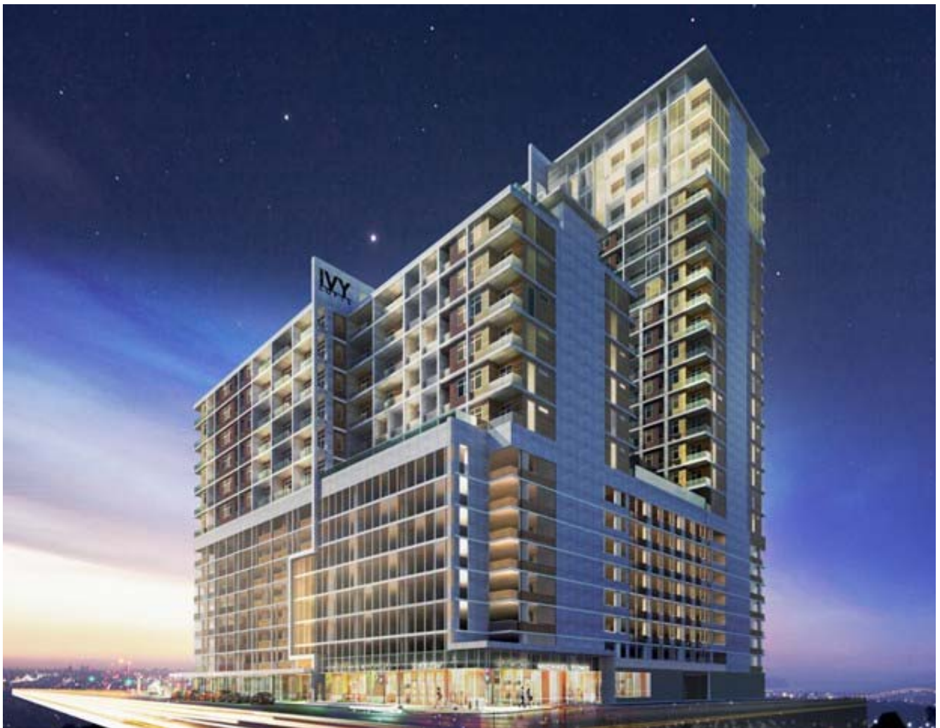
A multifamily development in Houston that includes micro-units lords over space. (Novel Creative Development)
