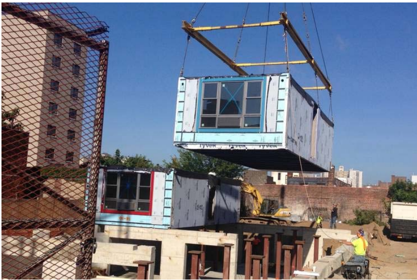
A crane lowers a module into place. PHOTO: JAMES MCCULLAR ARCHITECTURE
